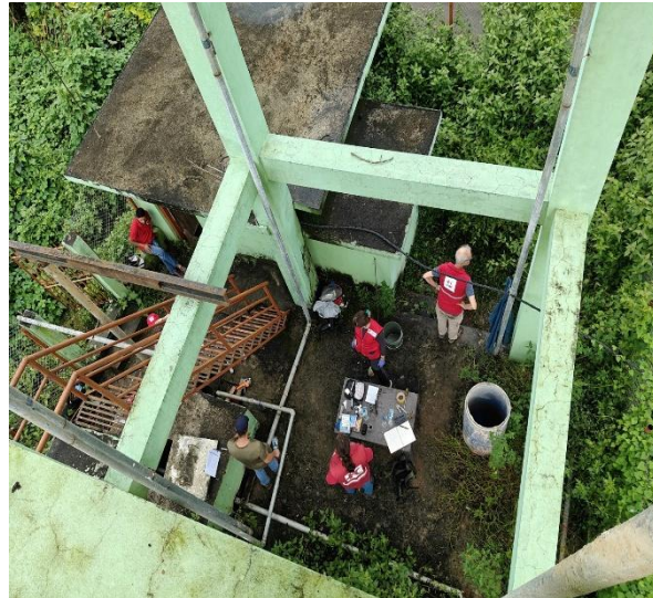
Photo: Borehole testing and water quality testing of Maharanihi water supply system-Bidhur Municipality-6 for overall rehabilitation of the system
