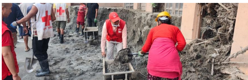
Photo: NRCS volunteer supports in debris clearance, Dhading
