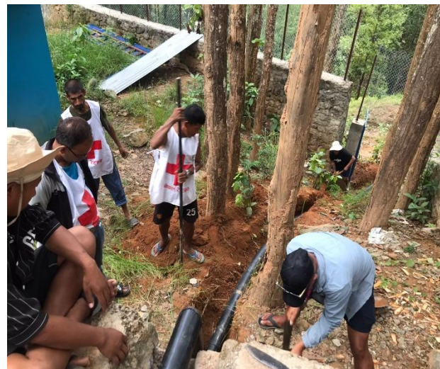
Photo: NRCS supports reconstruction and repair of water supply system in flood affected area at Betrawati
