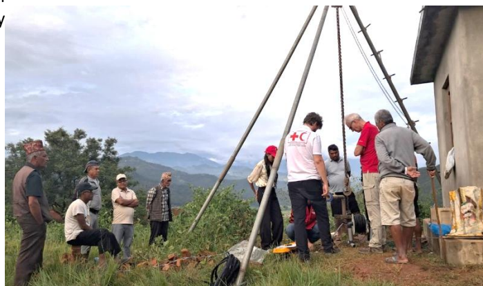
Photo: NRCS supports reconstruction and repair of water supply system in flood affected area
